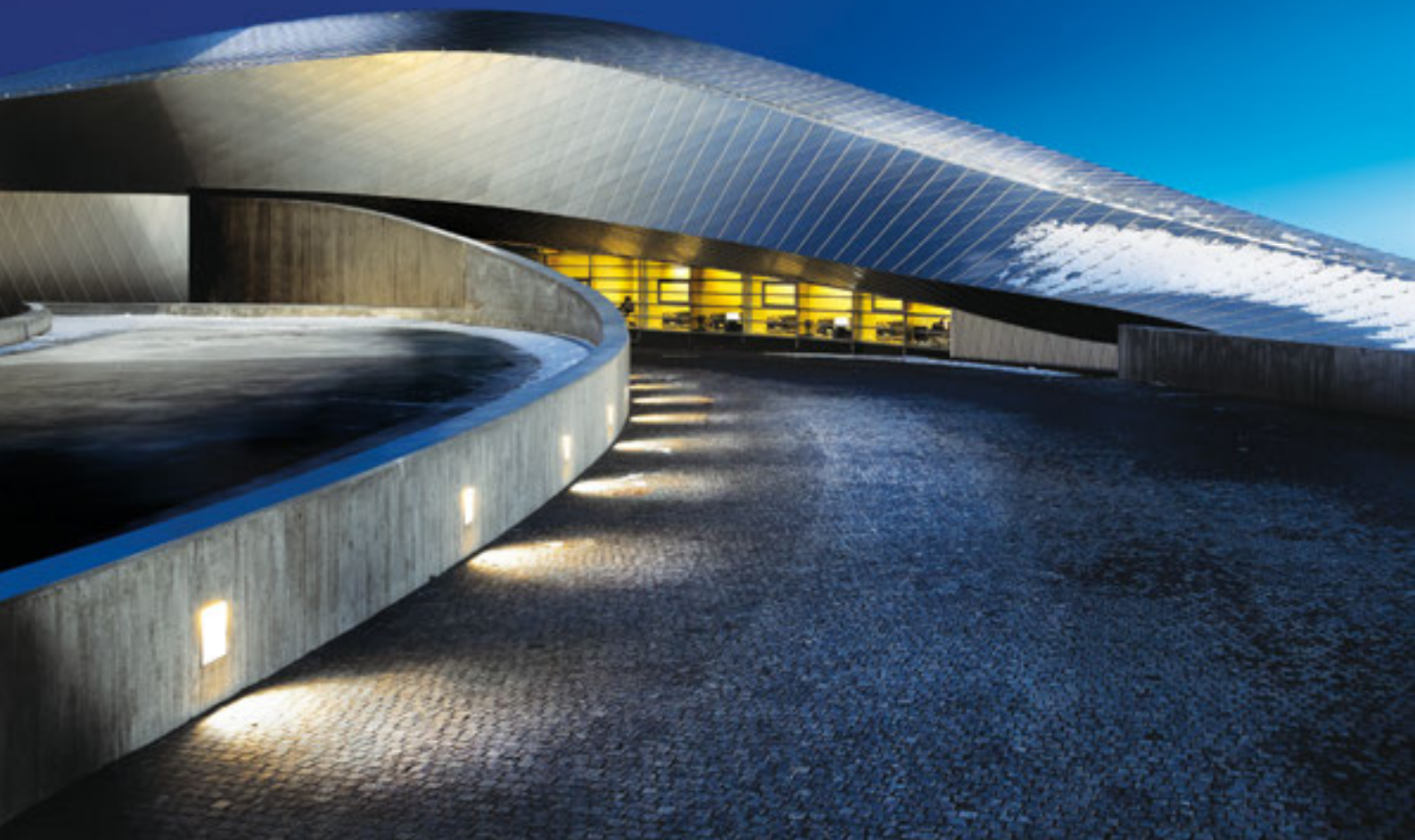
The Blue Planet Building Foundation, Kastrup, Denmark - Arch. 3XN © ph. Tom Jersø
