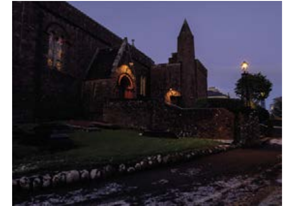
After lighting intervention
